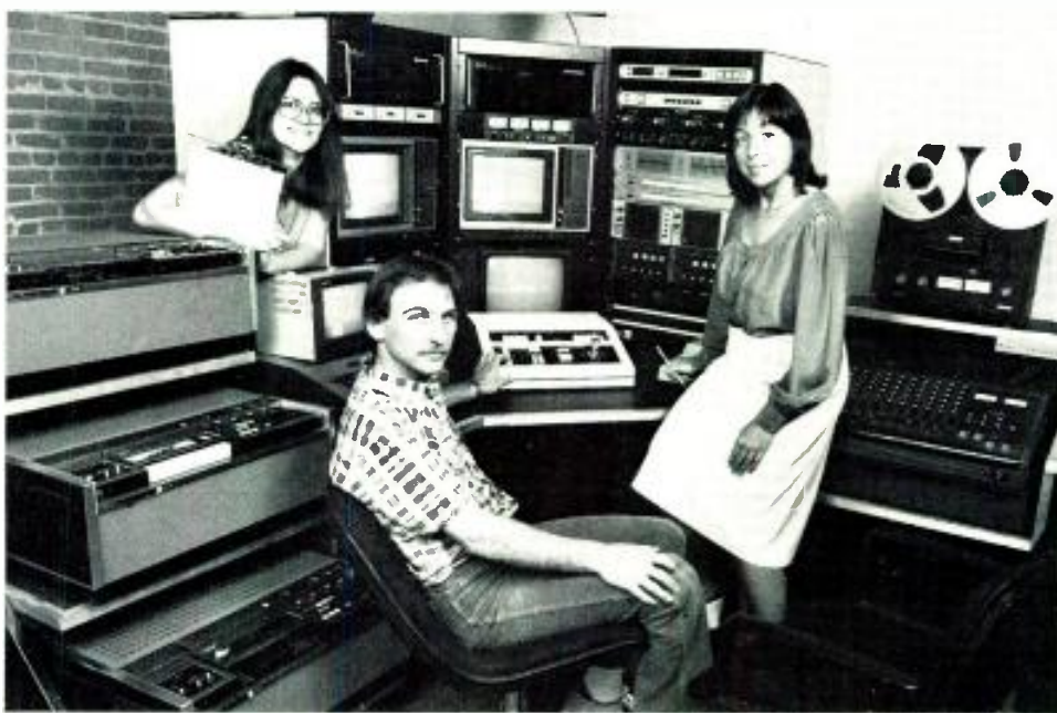
Equipment in the second of Varitel's two 3/4-inch edit suites includes (left to right): three BVU-200s, Microgen character generator, Convergence 103B editor, Texas Instruments printer, Gray time code generator and reader, UREI 565 notch filter and 535 graphic equalizer, Adda VW1 remotes, Yamaha power amp, JBL and Auratone monitor speakers, Otari MX 5050 ATR, Yamaha 12 x 2 audio console, and Technics turntable.
